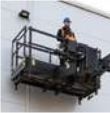
Man platform ready
